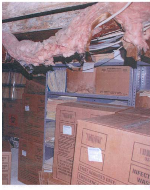
Boxes of bio-hazardous waste in basement
