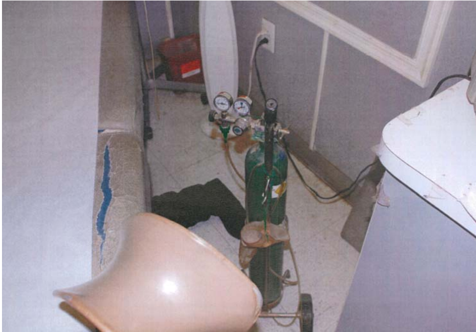
Procedure room, depicting ripped procedure table & stirrup, dust-covered oxygen tank, corroded tubing,
